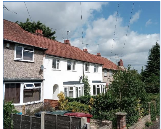
377 & 379 Norcot Road Site Photo taken on 18/08/2021
